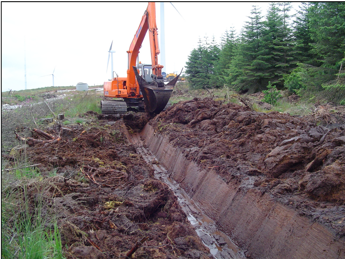
Plate 5. Cable trenching in progress
