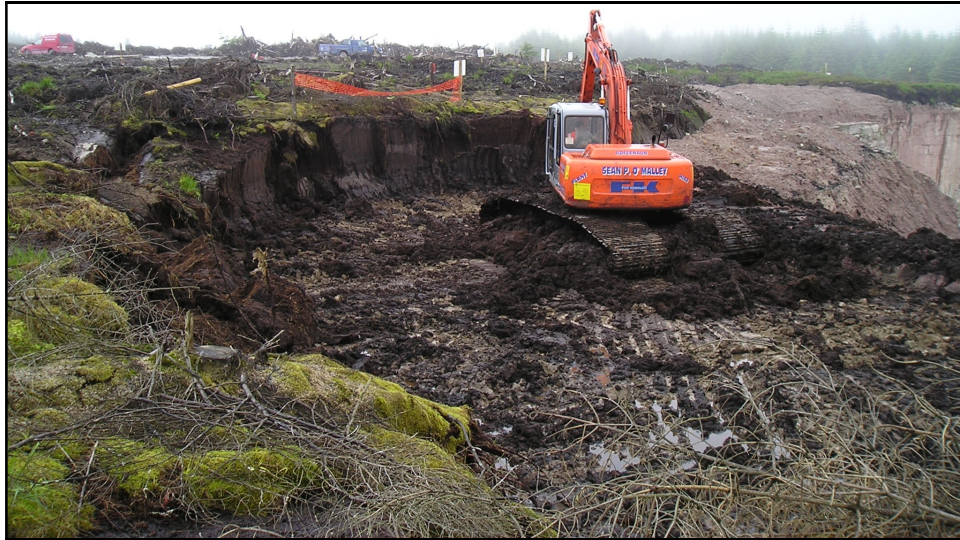
Plate 1. Mechanical excavator removing peat
