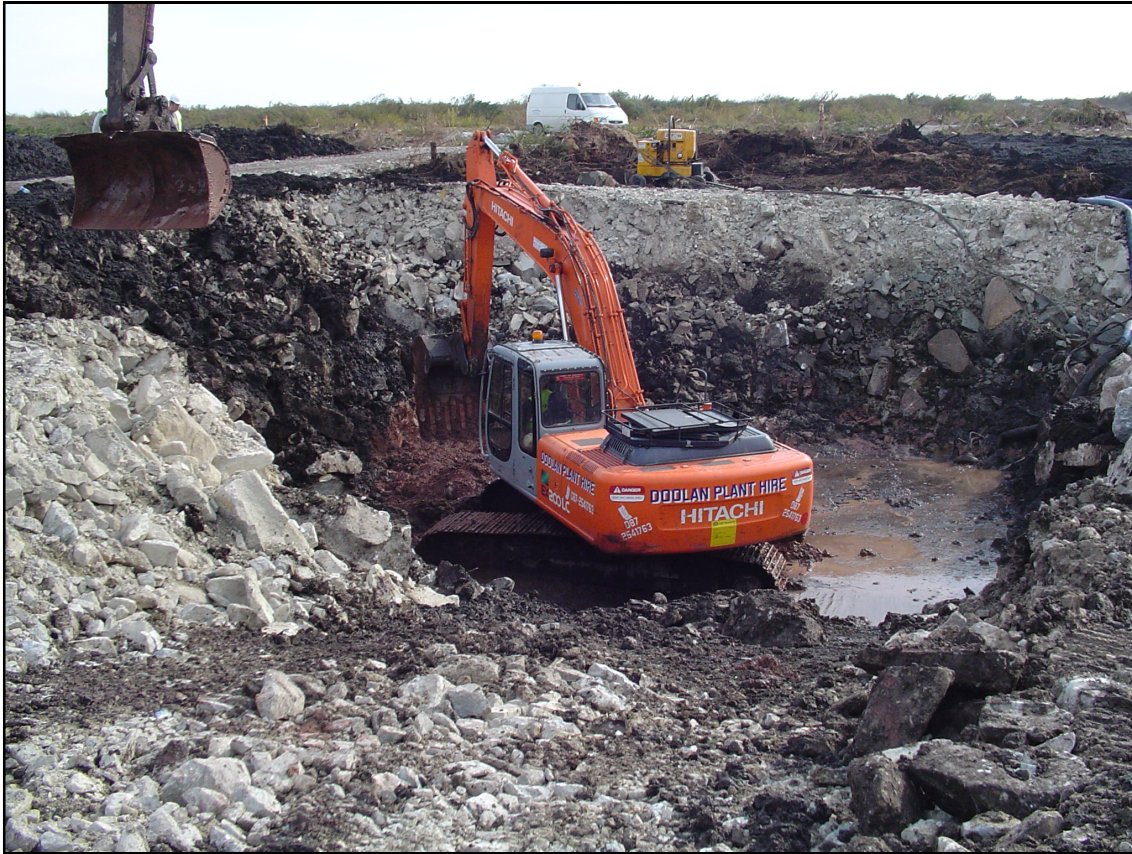
Plate 3. Stone crane base and excavated turbine base
