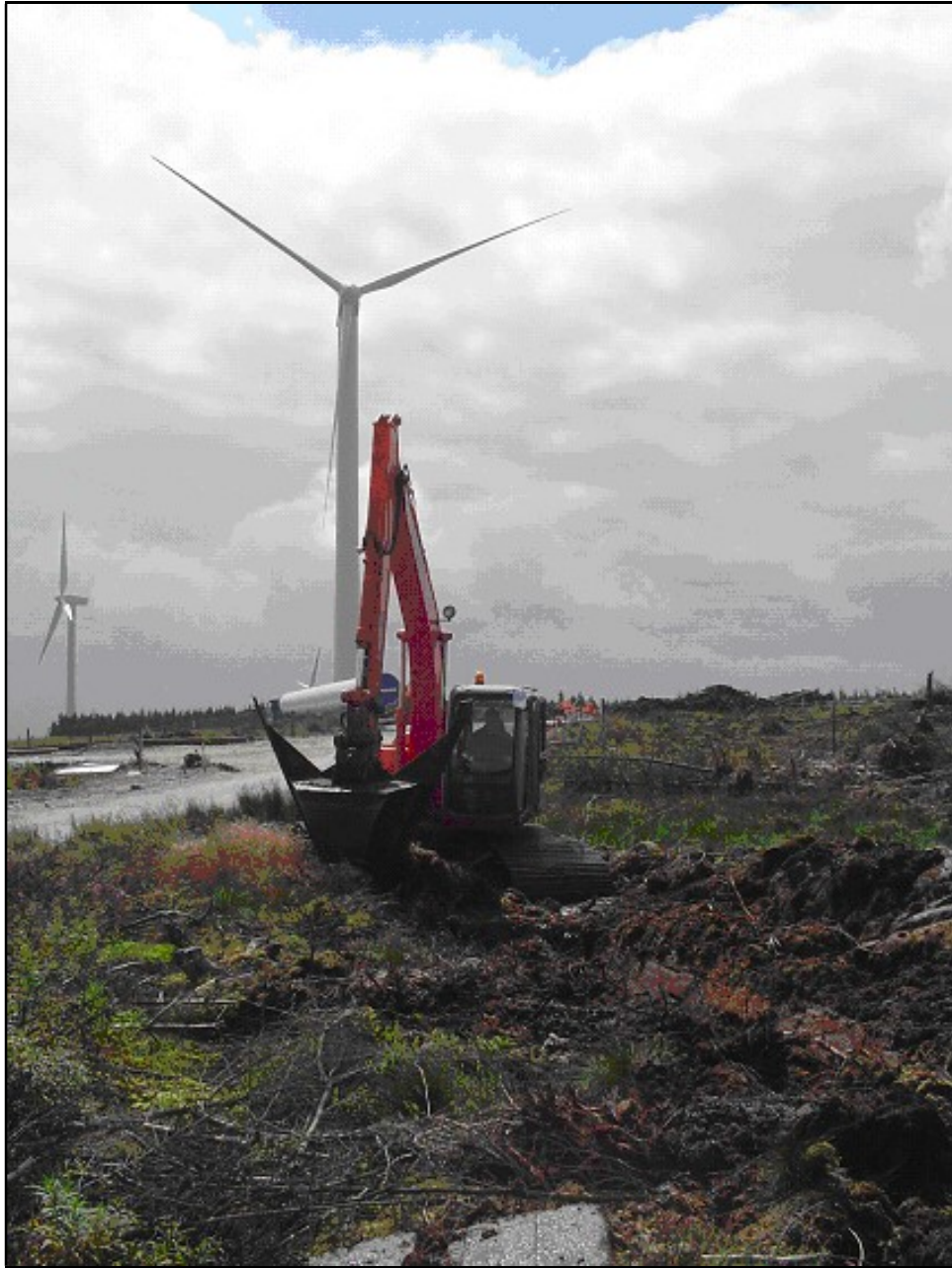
Plate 6. Cable trenching towards a nearby wind turbine
