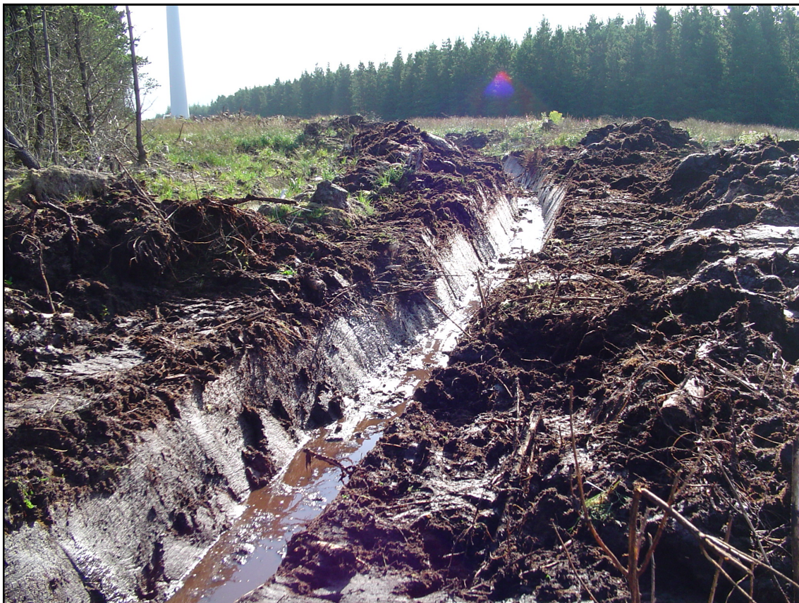
Plate 8. Excavated cable trench
