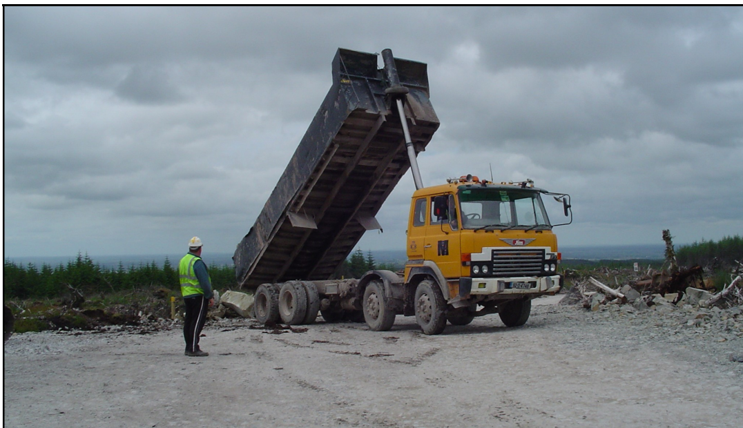
Plate 2. Lorry depositing rock after peat removal
